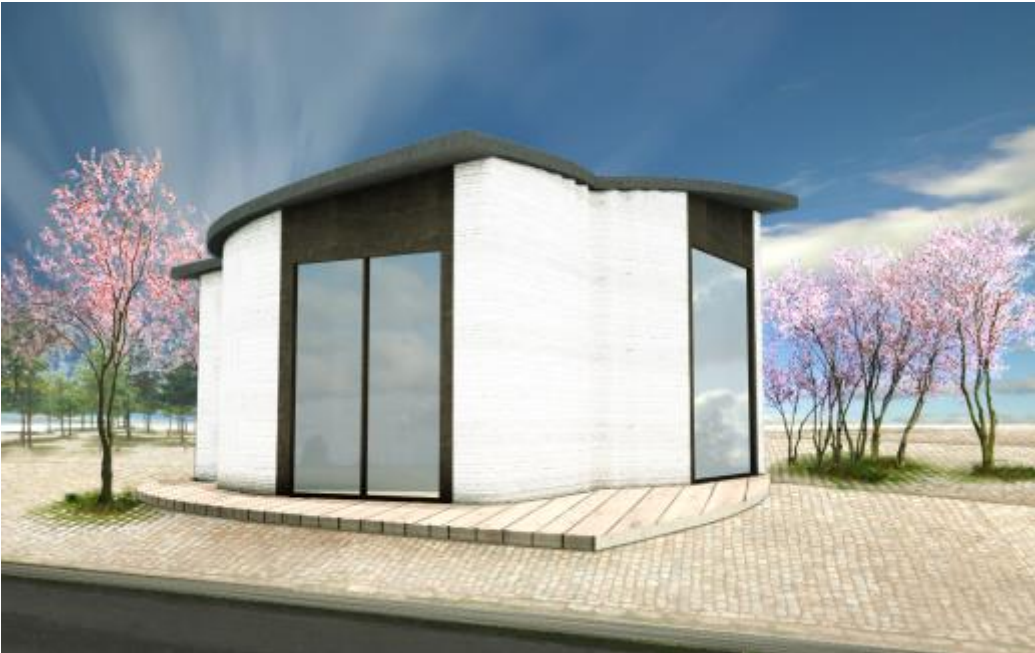
The BOD (“Building on Demand”) building in Copenhagen Harbour with curved 3d printed walls and sloped roof (Architect Ana Goidea, MAA)
