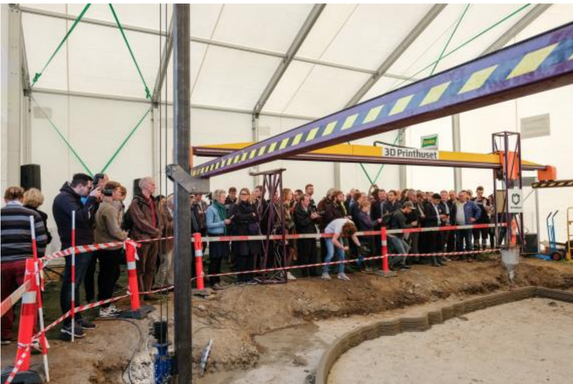
Inside the tent, the attendees were studying live 3D printing of The Bod – Europe's first 3D printed building.
